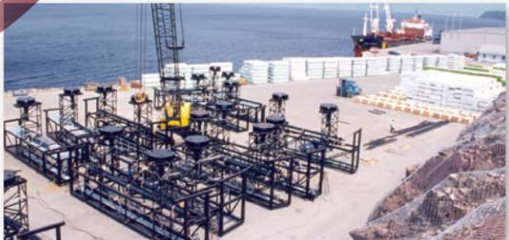
Oil distribution module • Newfoundland, Canada
